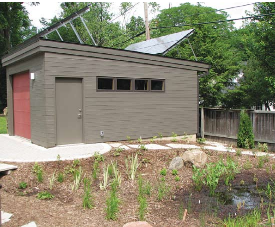
Solar panels on the detached garage and water retention with native plants.
